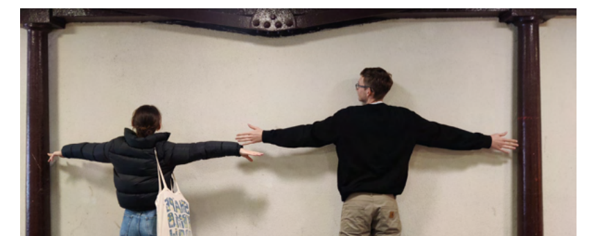
Measuring the underpass columns (next time bring a tape measure...)
